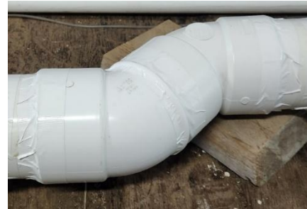
Figure (30): Six inch angled 45 degree offset pipe fittings
