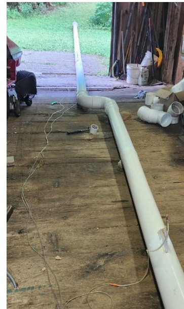
Figure (29): Six-inch 90 degree sweep offset fittings
