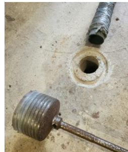
Figure (14): 2.5" core enlarged to 5" core
